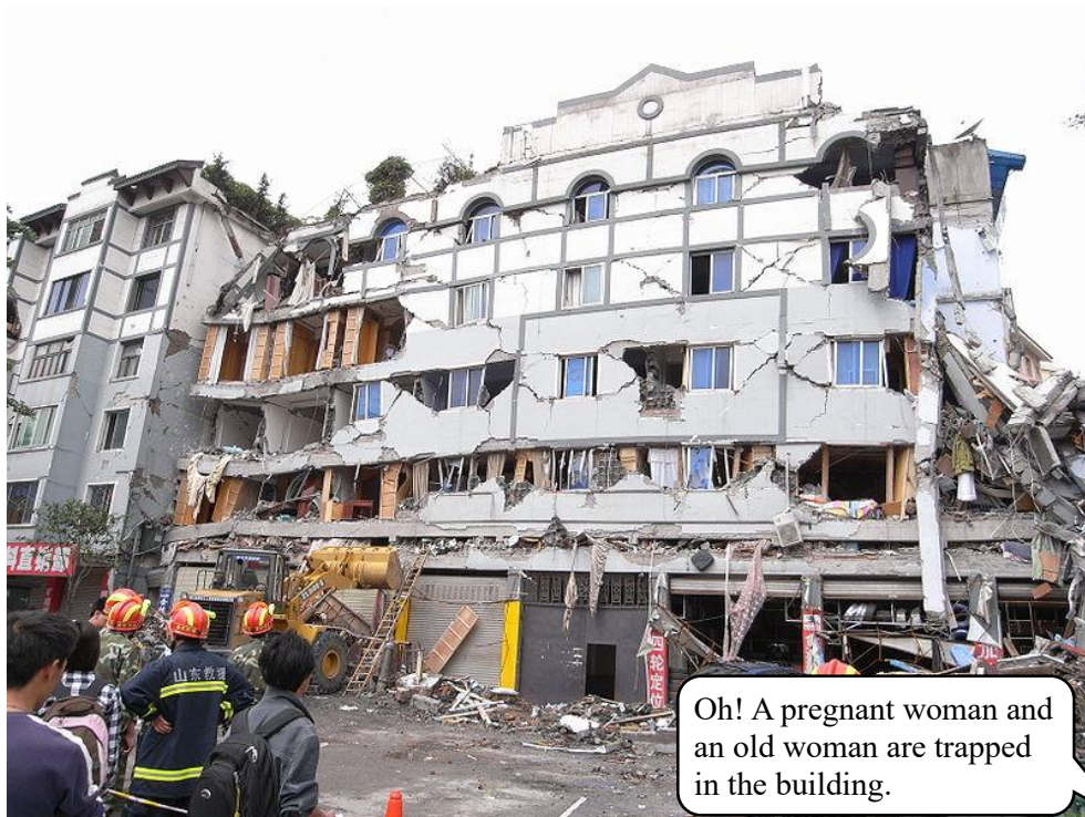
A building collapsed in the Sichuan Earthquake
